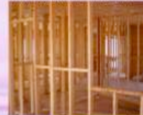
Timber for house constructions
